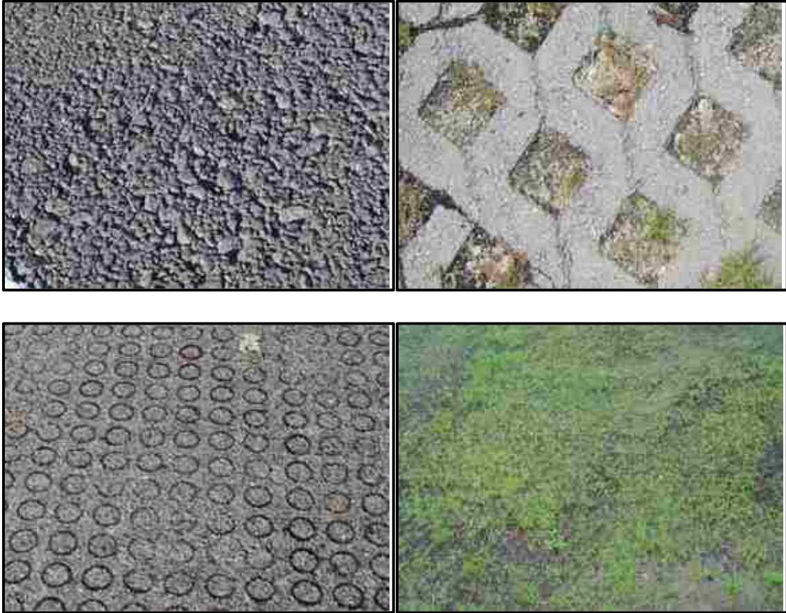
Figure 2.6-1: Porous asphalt (top left corner); Concrete grid pavers (top right corner); Gravel pavers (bottom left corner) and Grass pavers (bottom right corner) (Hunt and Collins, 2008)
